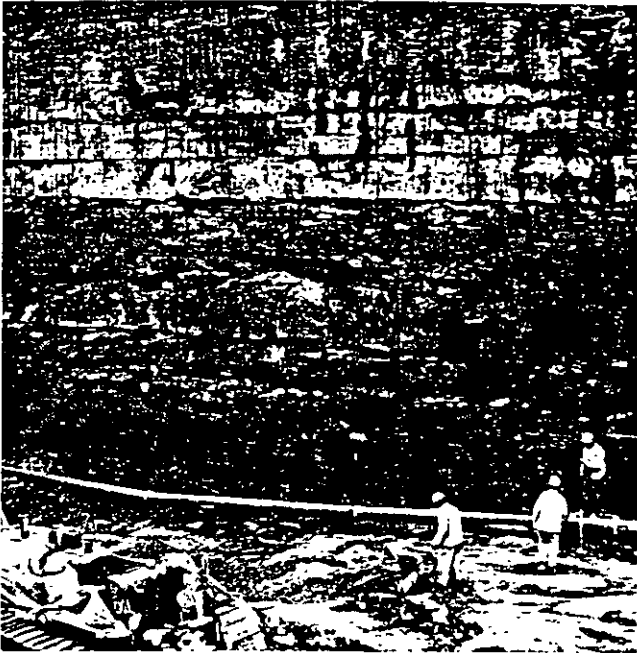
PRE-SHEAR RESULTS IN HIGHLY STRATIFIED FORMATIONS
