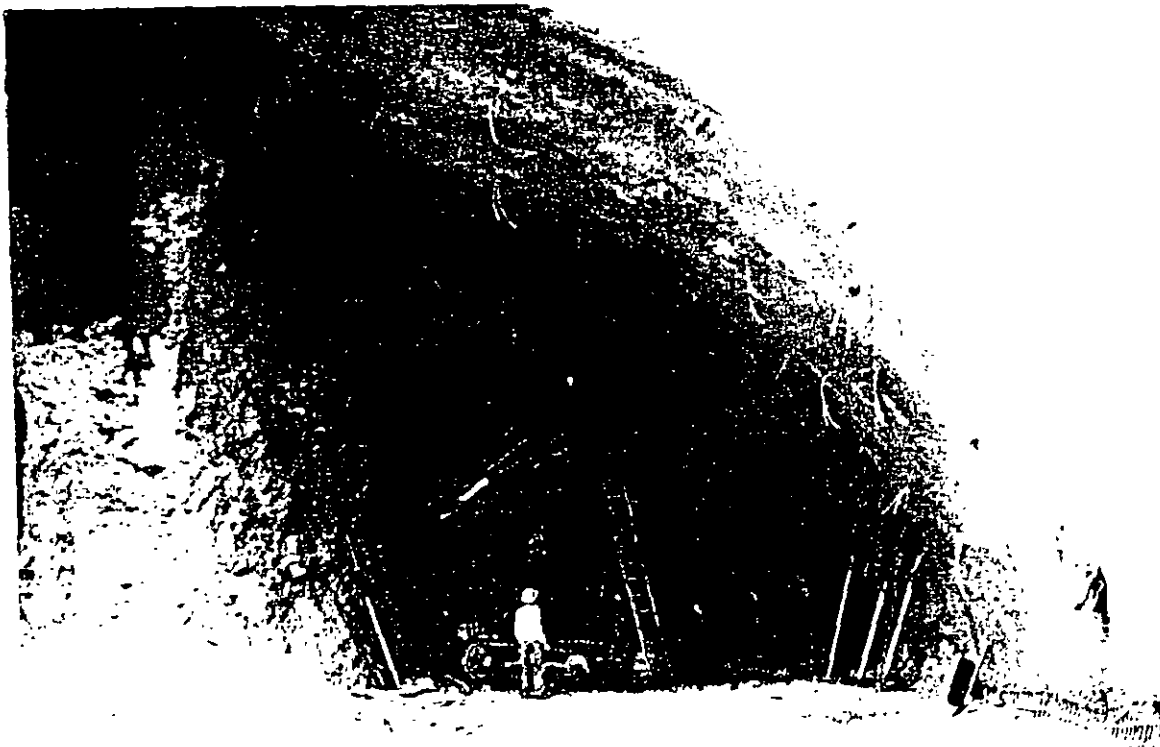
Progress of Side Tunnel
