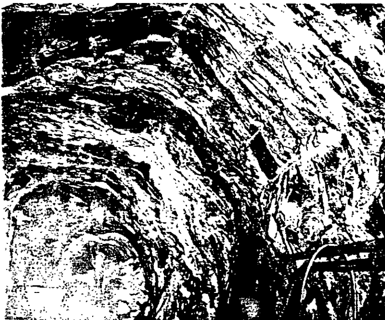
SMOOTH BLASTING RESULTS IN UNDERGROUND HEADING
