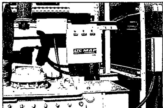
figure 5. ECM IED installed on substation transformer
