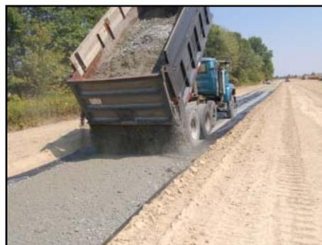
**FIG. 3.28 DESCARGA DEL MATERIAL GRANULAR SOBRE LA GEOMALLA**
