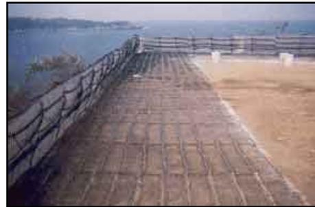
FIG. 3.16 GEOMALLAS MONO-ORIENTADAS, SUJETAS A LA CIMBRA Y AL SUELO
