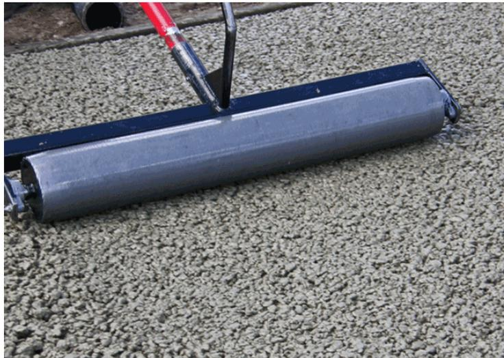
Figura 4.8 Rodillo pequeño usado para compactar una área pavimentada pequeña ([http://www.perviousconcrete.com/images/build07/cert\\_pervious\\_roller.gif](http://www.perviousconcrete.com/images/build07/cert_pervious_roller.gif)).
