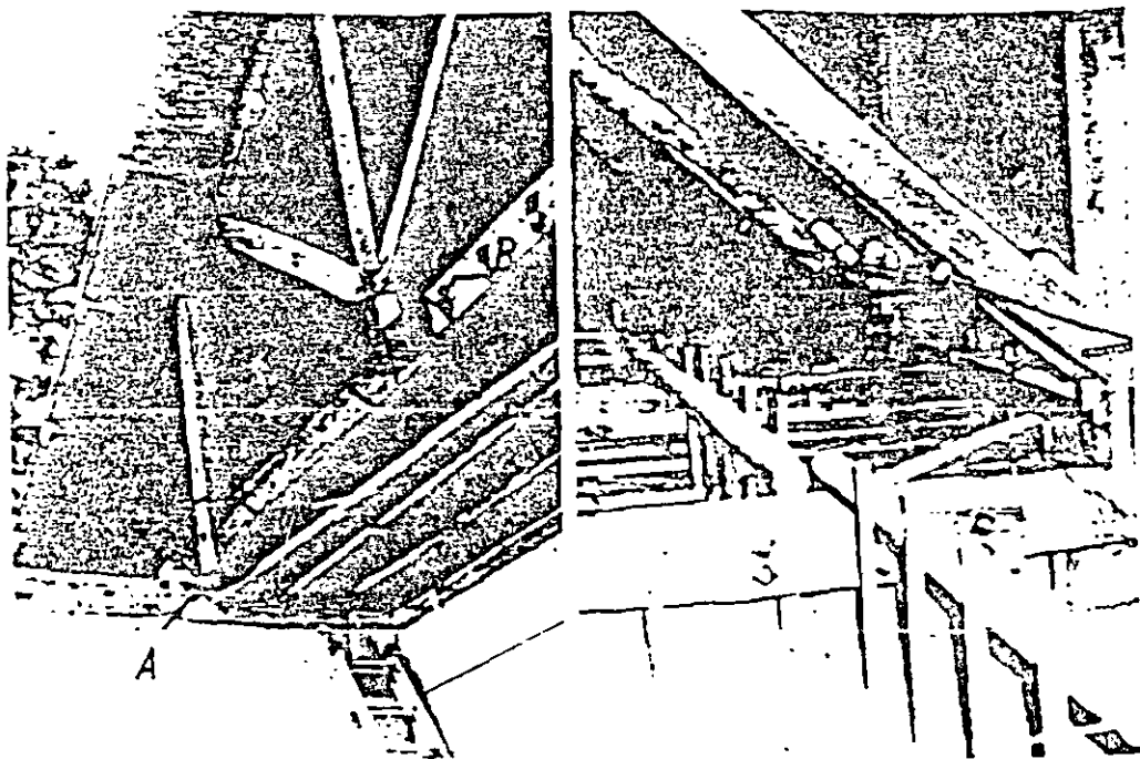
Fig. 2-71. Example of wooden king post truss
