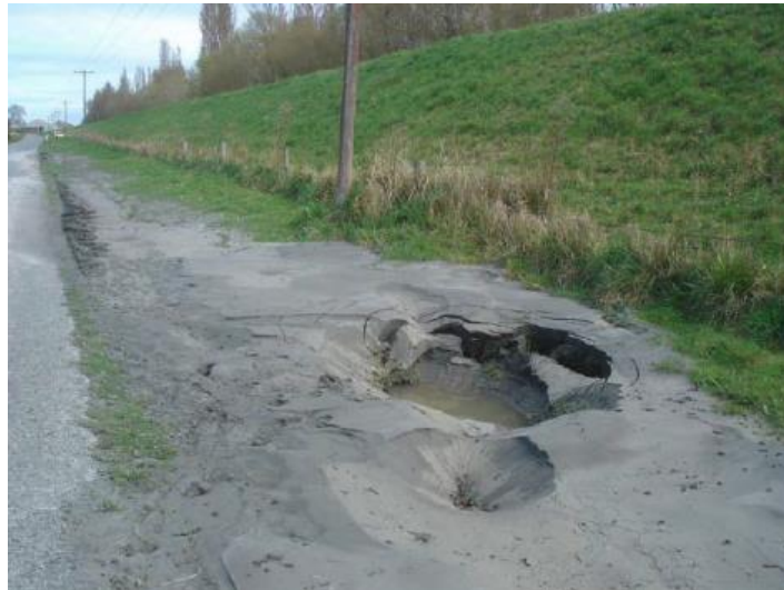
Fig 1.3 Gran volcán de arena en la base de una ladera (Geo-engineering Extreme Events Reconnaissance Association [GEER Association], 2010c)
