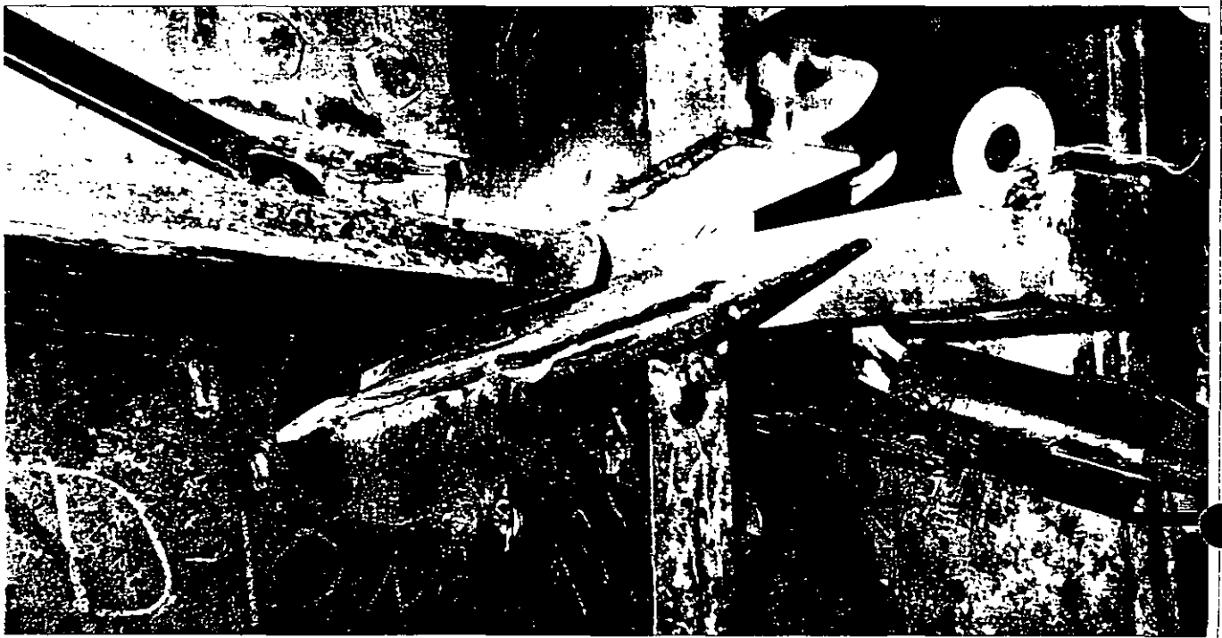
A CRACKED COLUMN FLANGE IS PREPARED FOR WELDING AFTER REMOVAL OF A CRACKED SECTION.
