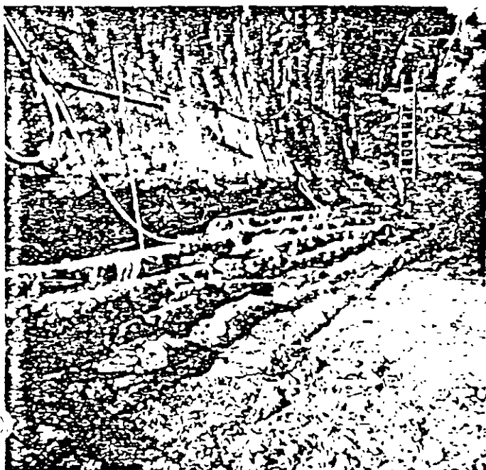
Fig. 33. Stages III and IIIa completed. Note the unsupported length of wall lining (about 20m). Below the wall lining the contact between clay and limestone can be seen
