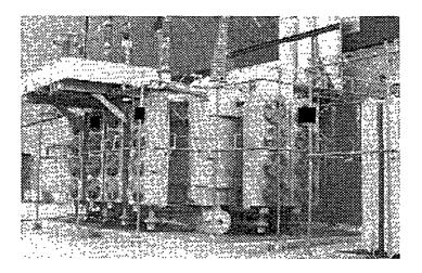
Figure 3 – Blocks indicates fans removed from service
