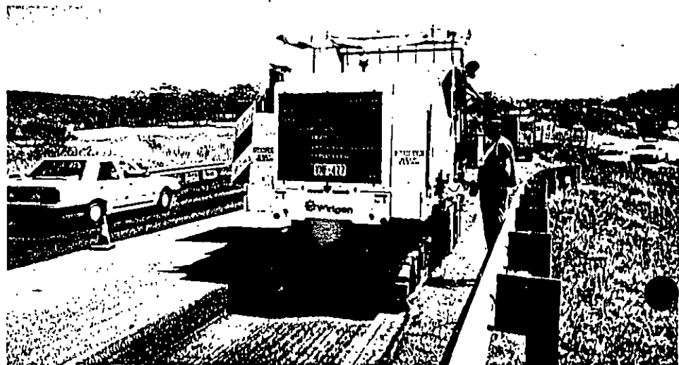
Wirtgen cold milling machines: Stripping and removing pavement in various working widths
