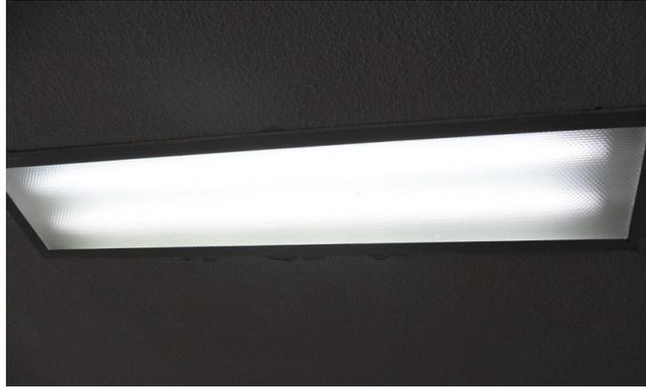
*Foto II.2 Luminaria fluorescente lineal T12 2x40 W*
