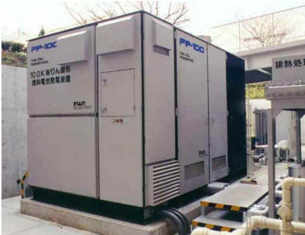
Fig. 2.5 Celda PAFC Fuji-Electric 100kw [7].
