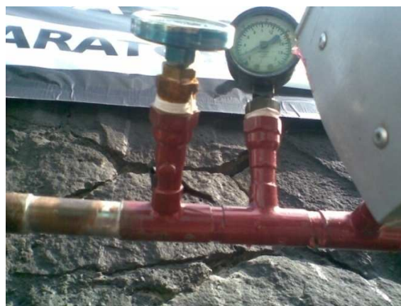
FIGURA 3.16. Colector Solar B.
