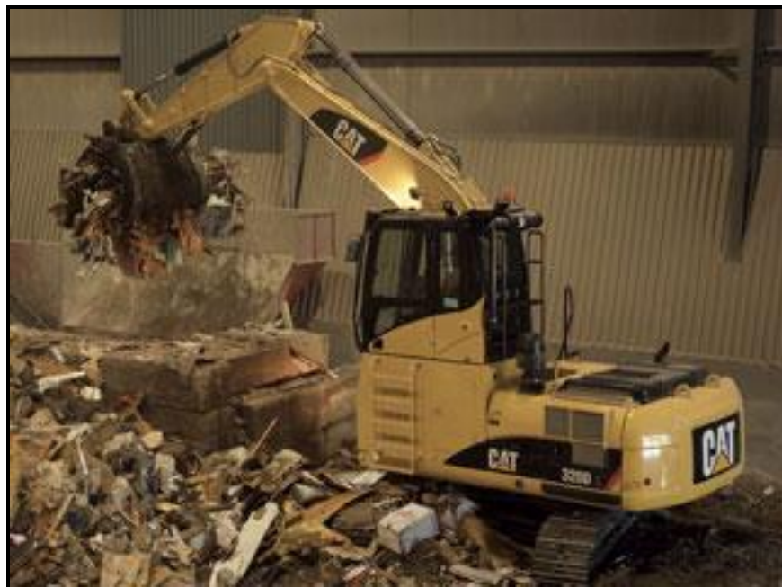
Figura 3.26 Grúa caterpillar (material handler).
