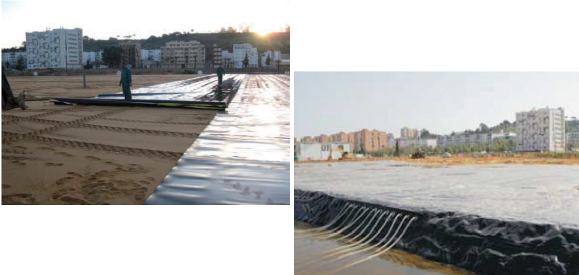
Figura 6.9.- Membrana impermeable (Menard, 2010)
