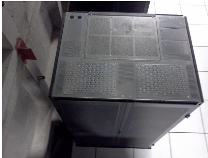
Fig. No. 19. PDU. 480 – 220 V. Emerson.
