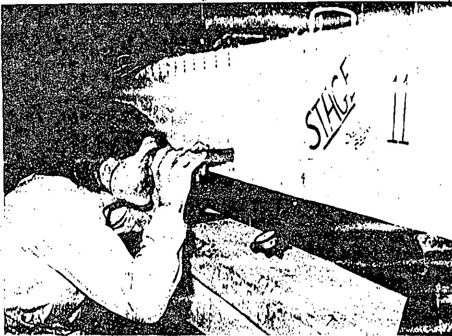
Photo 37 Simply supported beam prior to developing diagonal tension crack (load stage 11). (Test by Nawy et al.)
