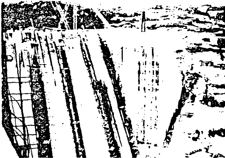
Figure 9.17 Gravity block required for the upper part of the right abutment of Alto Rabagao Dam, Portugal. (Courtesy of Dr. Manuel Rocha.)
