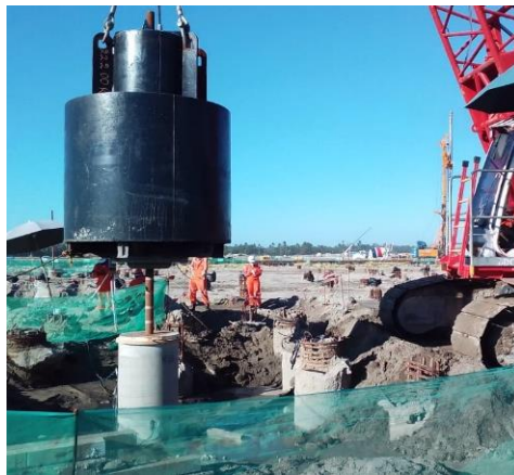
Figure 11. Dynamic load test system
