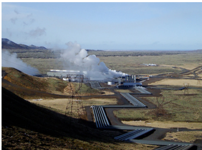
Figura 1.8 Central geotérmica en Islandia. (Creative Commons, 2010)
